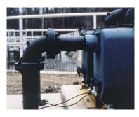
In this installation, two 3" Trash Hogs are being used to control the level of the liquid in these settling ponds. Liquid level controls in the sump determine whether either or both pumps are needed to maintain proper pond level. Trash Hogs were chosen due to their reliable priming capabilities.
