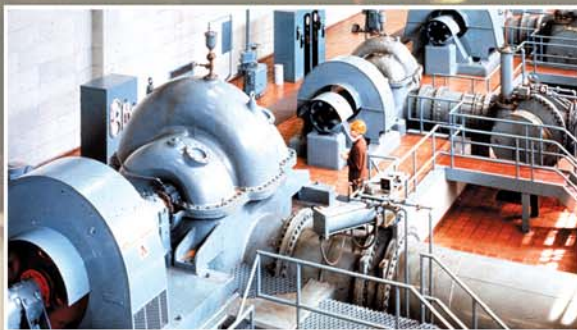
Goulds split case pumps have many applications in the power generation market.
